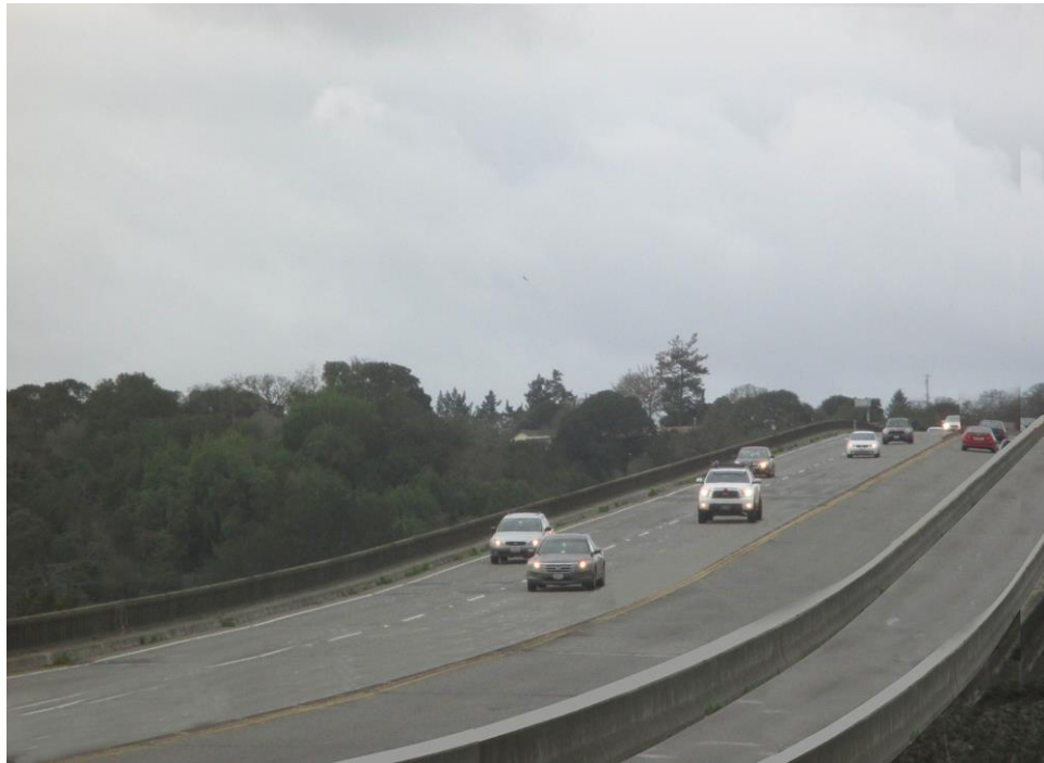
Simulated bypass image based on 65 foot wide bridge as described in Alt. 1 from the Air Quality Appendix of the DEIR/S; from Jim Sajdak
