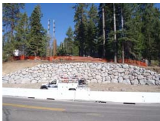
Rockery wall on SR 89 across from the Caltrans Maintenance Yard. The Williamson Tree will be relocated above the rockery wall.
