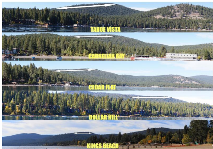
Location of ridgeline from multiple in-Basin locations. Image prepared by GK Consulting View larger image
