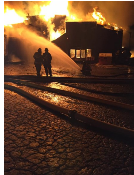
The 12/28 fire at the South Lodge. (Source: Sierra Sun )
